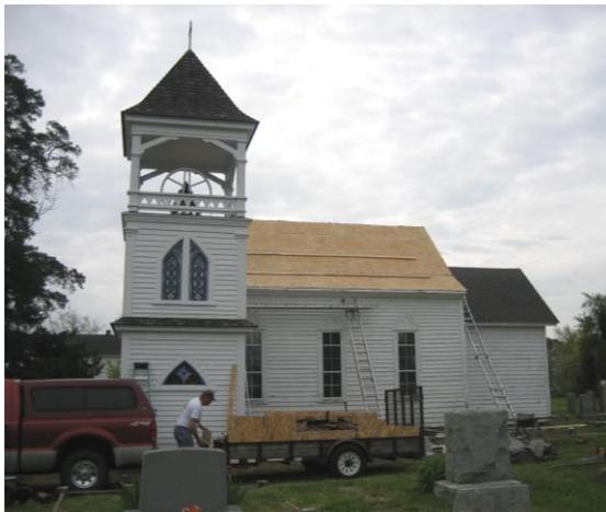
right half of the main church. The wooden cross on top was repainted and the old furnace vent pipe was removed, making the roof more secure.
